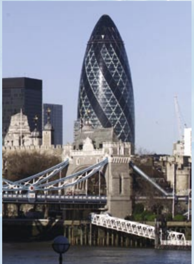
London's futuristic office building called 30 St Mary Axe is equipped with expertly engineered differential pressure regulators from SAMSON.
