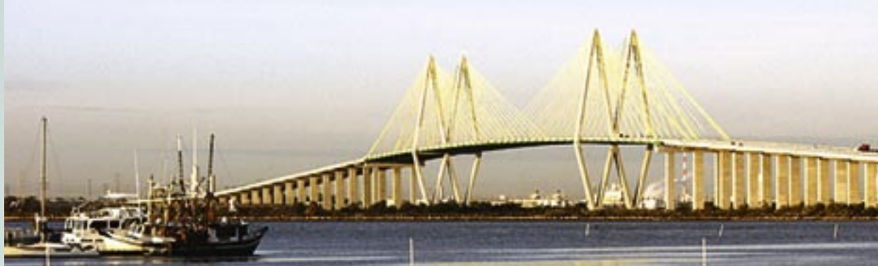
The graceful Fred Hartman Bridge, which connects the cities of Baytown and LaPorte, is a Texas landmark. The four-kilometer-long cable-stayed bridge crosses the Houston Ship Channel, one of Texas' transportation lifelines.
