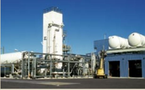
A helium liquefaction plant designed by Air Products. Liquefied helium at a temperature close to absolute zero is an excellent refrigerant.
