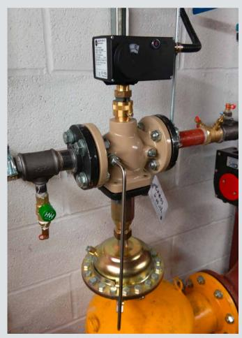
Fig. 3: Electric control valve with flow regulator to control the primary bypass
